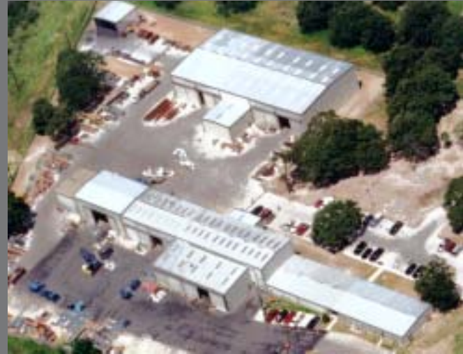
DYNACON's Bryan, Texas, U.S.A. facility
